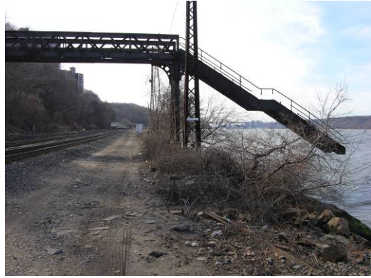
Remnants of bridge to water at 231st Street
