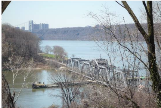
Spuyten Dyuivil Bridge from Kappock Street
