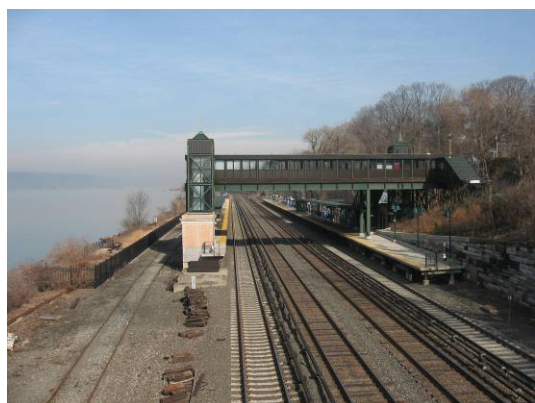
Riverdale Station from 254 th Street
