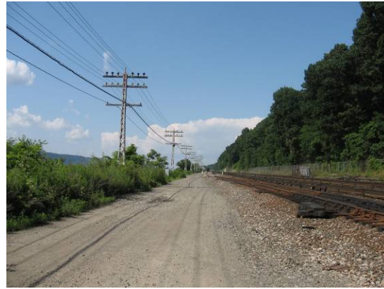
Maintenance road between waterfront and tracks
