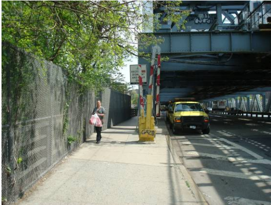
Broadway Bridge walkway
