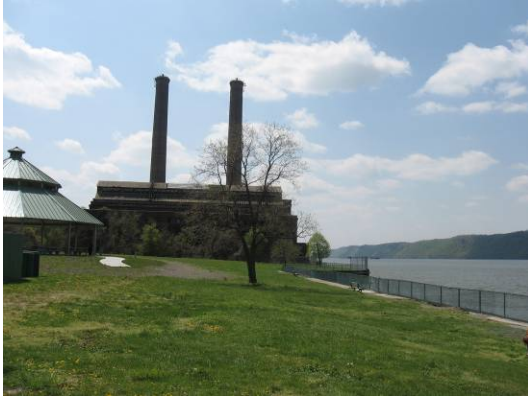
Glenwood Power Station
