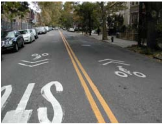
Pavement markings along Tibbett Avenue
