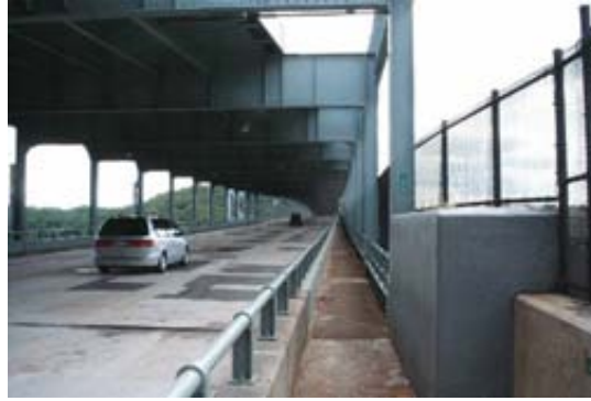
Henry Hudson Bridge walkway
