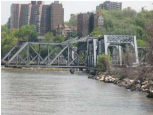
Spuyten Duyvil Railroad Bridge
