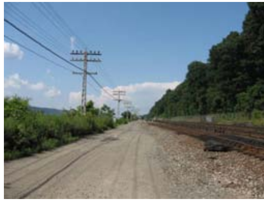
Maintenance road between waterfront and tracks
