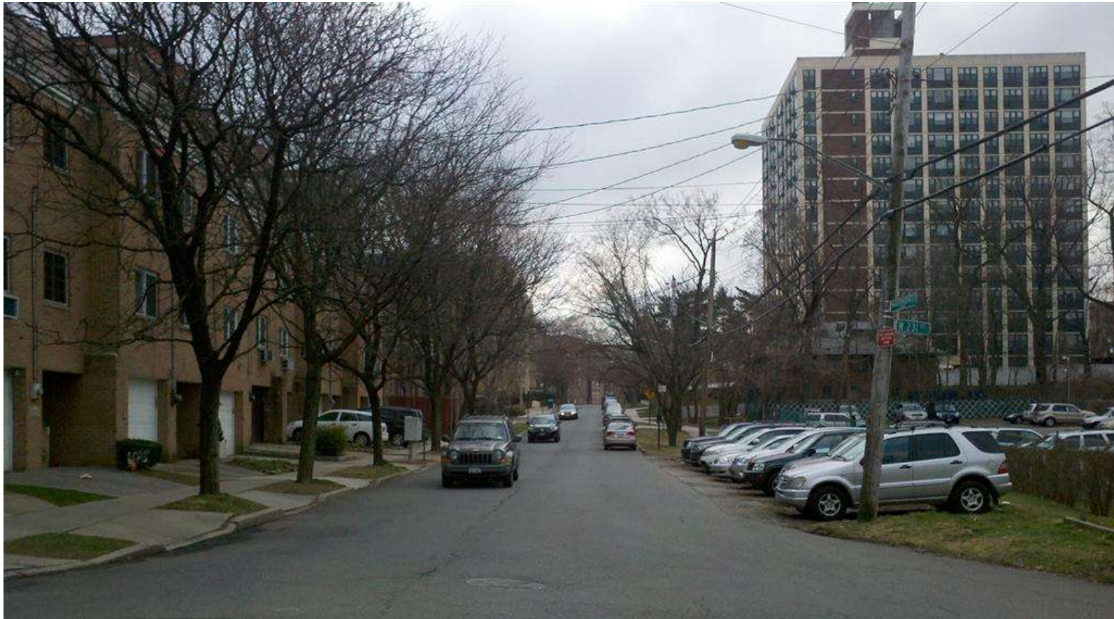
EXISTING CONDITIONS – Independence South of 231st St
