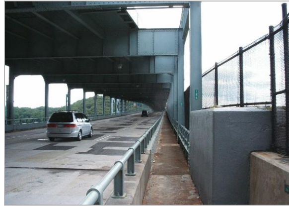
Figure 2: Henry Hudson Bridge Lower Walkway
