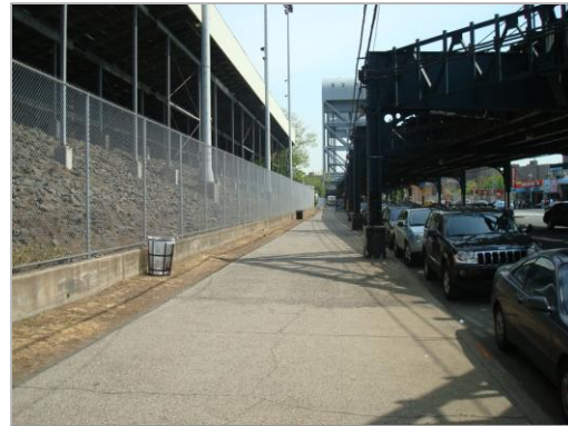
Figure 6: Sidewalk on West Side of Broadway between 218 th Street and Broadway Bridge
