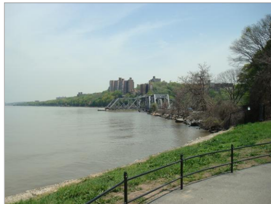
Figure 8: Railroad Swing Bridge at Spuyten Duyvil view from northern end of Inwood Hill Park at the Hudson River
