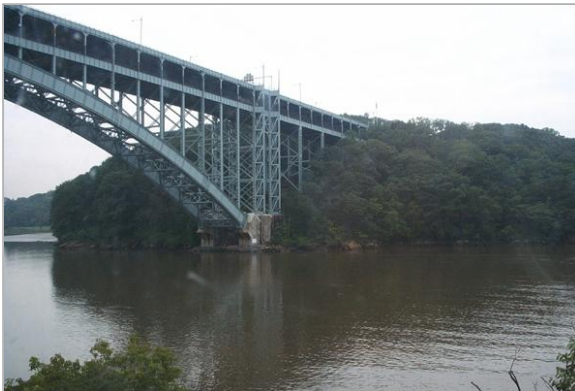
Figure 3: Henry Hudson Bridge
