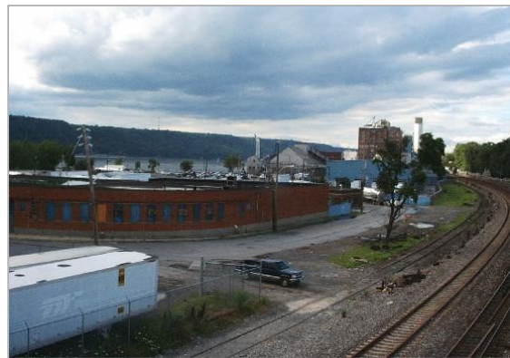
Figure 19: Industrial uses along the Yonkers waterfront
