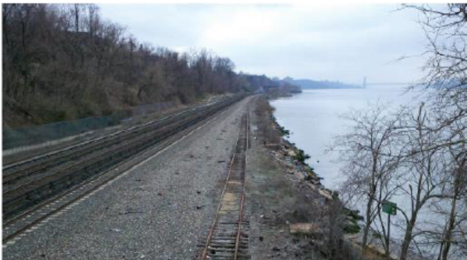
View Looking South along Hudson River Shoreline from College Point Bridge
