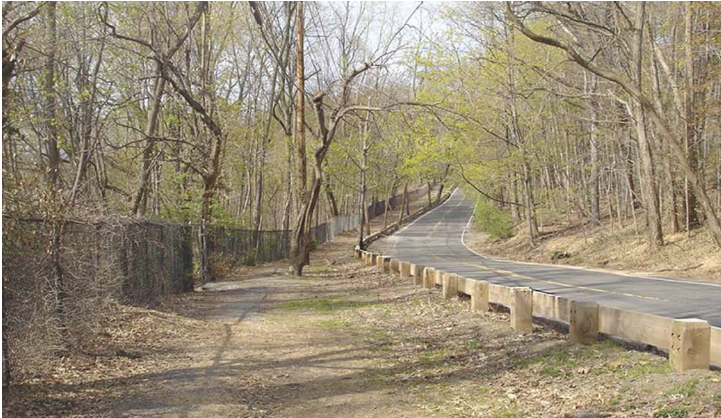
Existing Photo Palisades Avenue - BEFORE
