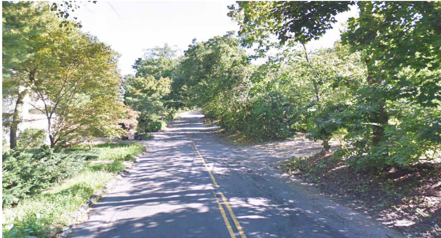
Palisade Avenue north of 254th Street
