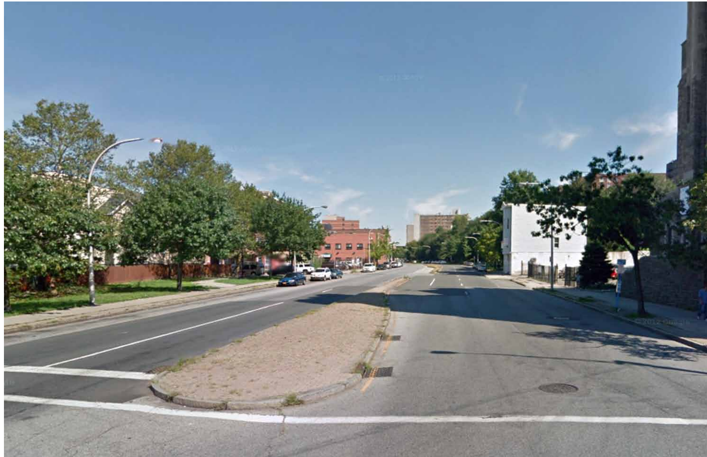
Riverdale Avenue at Ludlow Street Facing North
