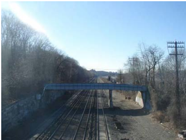
Existing maintenance road adjacent to tracks
