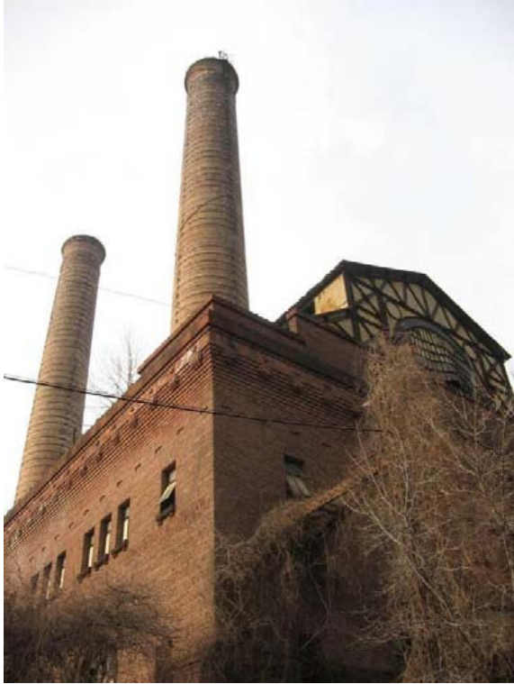
Abandoned Glenwood Power Plant
