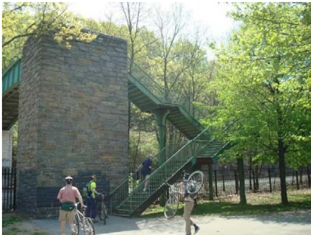
Stairs leading to bridge over tracks in Inwood Hill Park
