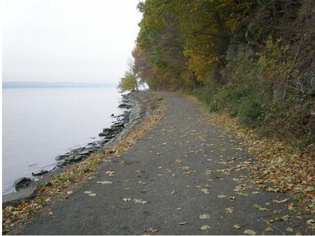
Stabilized Stone Screening on path in Nyack Beach State Park
