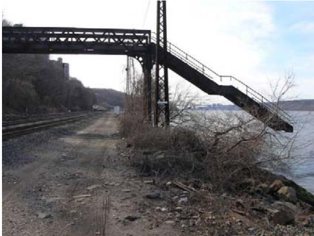
Maintenance road, scrubby vegetation, rip rap, ballast and bridge remnants
