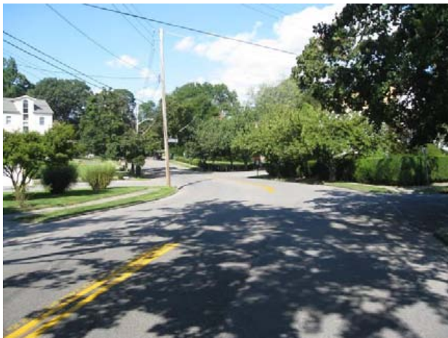
Sunnyside Drive between Valentine and Pier Street
