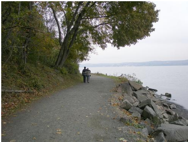
Stabilized stone screening as seen in Nyack State Park
