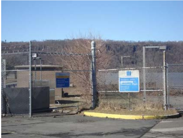
Gated entrance to the Westchester County Wastewater Treatment Plant
