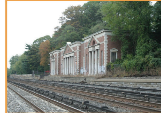
Historic Waste Treatment Plant
